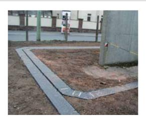
Municipal utilities Trier: Wiring of a transformer station with Vario Tec+ size 2.
