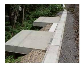
Custom solution: Excess cable kit with sand covered lids.
