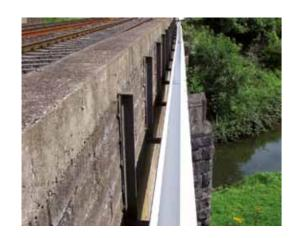
Custom solution: Vario Top size 1a is directly attached to a bridge with the help of special mounting brackets.
