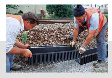
Installation of the ducts in the cable pits prepared beforehand.
