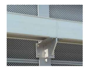
Vario Top size 2 mounted on special mounting brackets along a noise protection wall.
