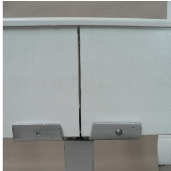
Image 6, use of grooved pin each 30m
