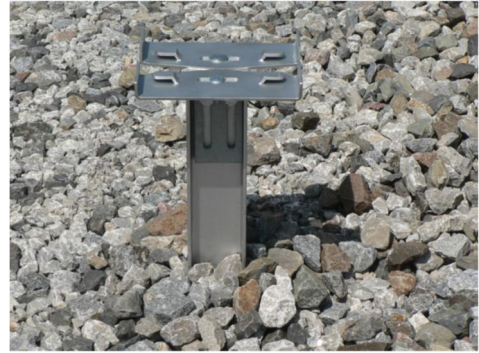
image 4, mounted fastening plate
